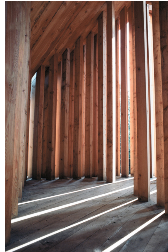
Structure poreuse Chapelle, Samuel Netocny Architects
